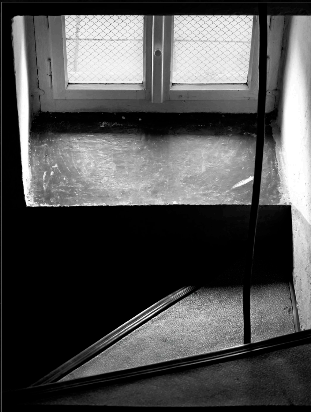
Cellar window, Germany
